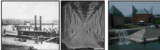
Civil War era steamer Civil War bridge Passage and Aquarium
